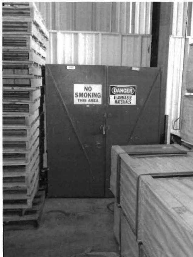
Photograph of Steel Storage Cabinet
